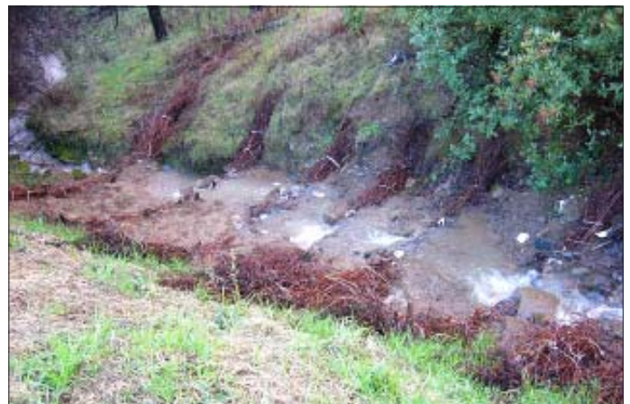
Willow Wattles reduce erosion in a gully recently cleared of garbage and replaced with native vegetation.
