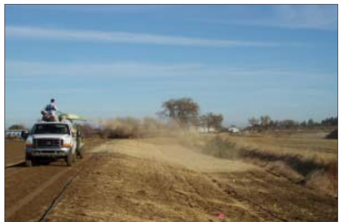
Audubon and NRCS staff blowing straw over the recently recontoured and seeded banks of Cottonwood Slough.
