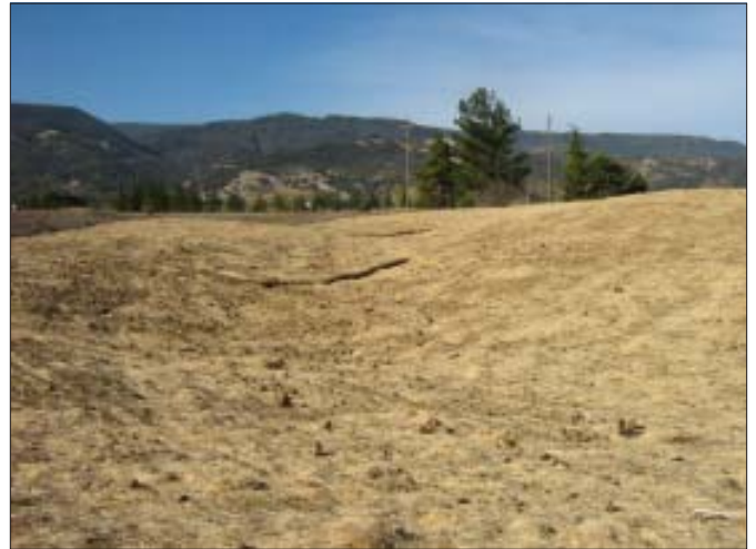
Cleanup site recontoured, seeded with native grass, and protected with straw wattles and native grass straw.
