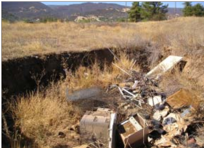
Cleanup site before garbage removal and gully repair.
