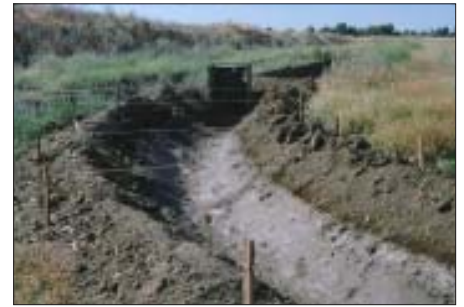
One of the elements of the study was to test sediment traps like this one. Results showed they capture a considerable amount of valuable soil.
